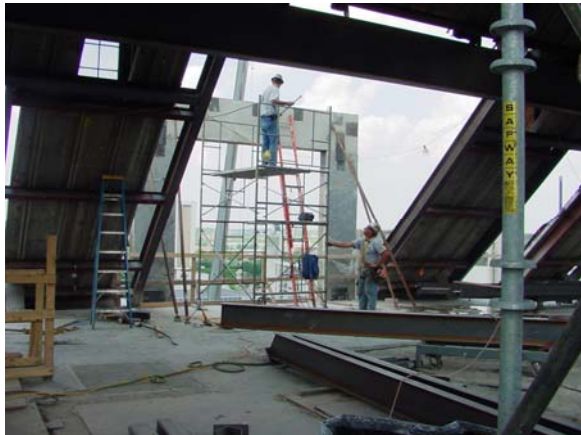
New Dormer added to Attic
