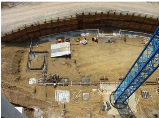
West Installation Basement Foundation
