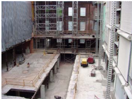
Interior of East Atrium looking North
