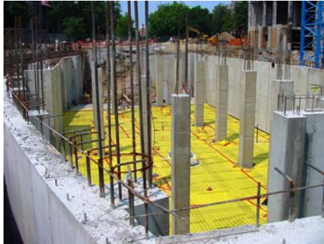
Basement Slab Prep
