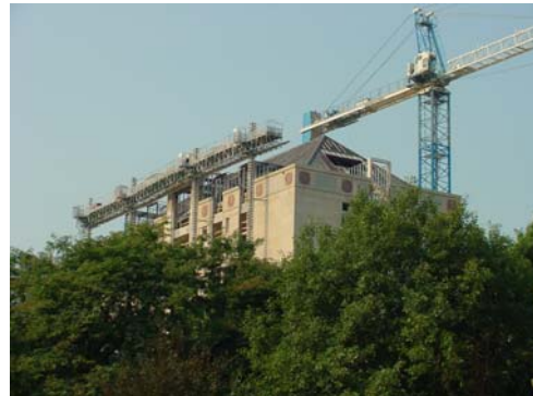
View of the Northeast Corner
