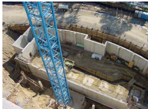
Foundation Walls for West Building Basement
