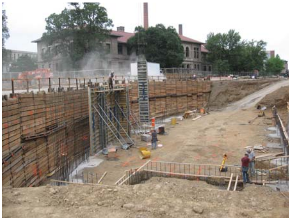
West Addition Basement
