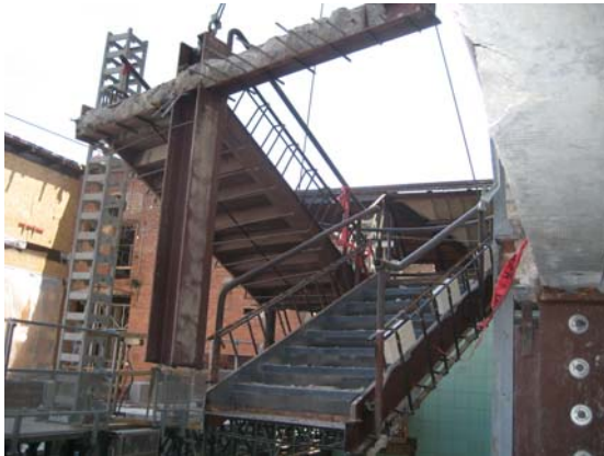
Level 2 Atrium Stair Removal By Crane
