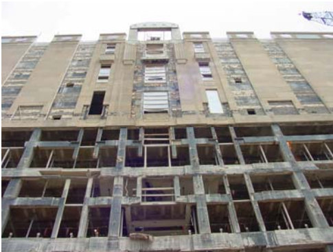
West Face Exposed - Level 3
