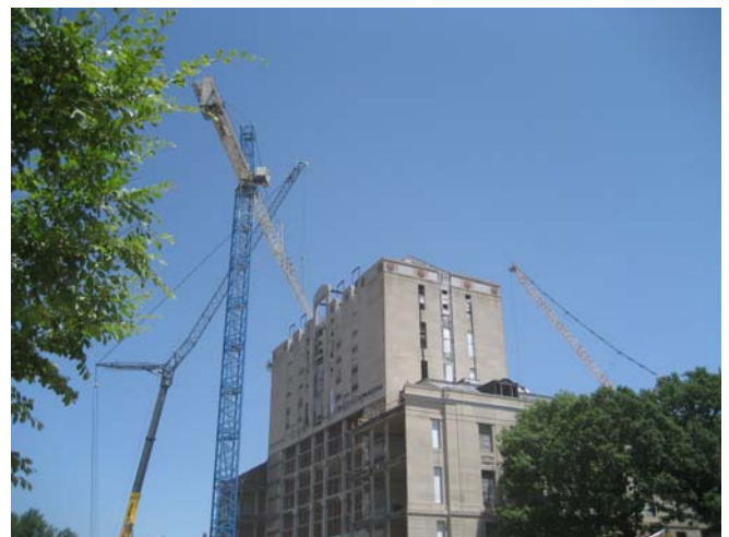
Cranes At Work
