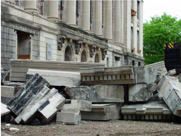
Cornice material from east Atrium
