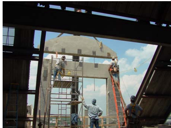
West Arch Re-Construction
