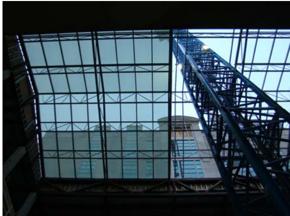
Looking up through the West Skylight Tower Crane still in place
