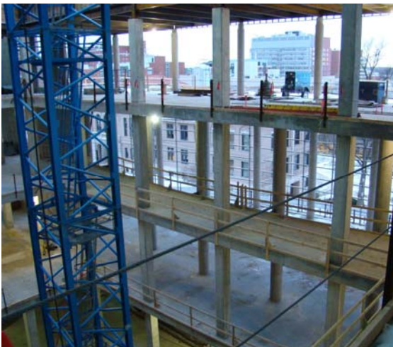
Looking southwest through the new West Building
